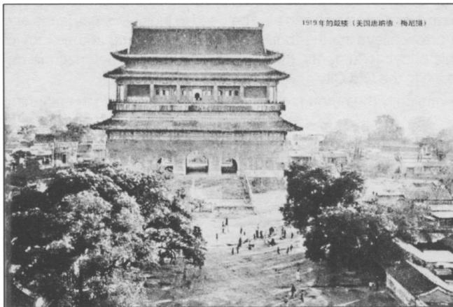
Fig. 5: Beijing Drum Tower in 1919, by Donald Meiny, US.
