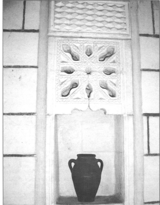
Fig. 2: A detail from the courtyard wall of an Antiochia house which has a niche which differentiates in usage according to different cultures. (Source: Yilmaz, 2004).
