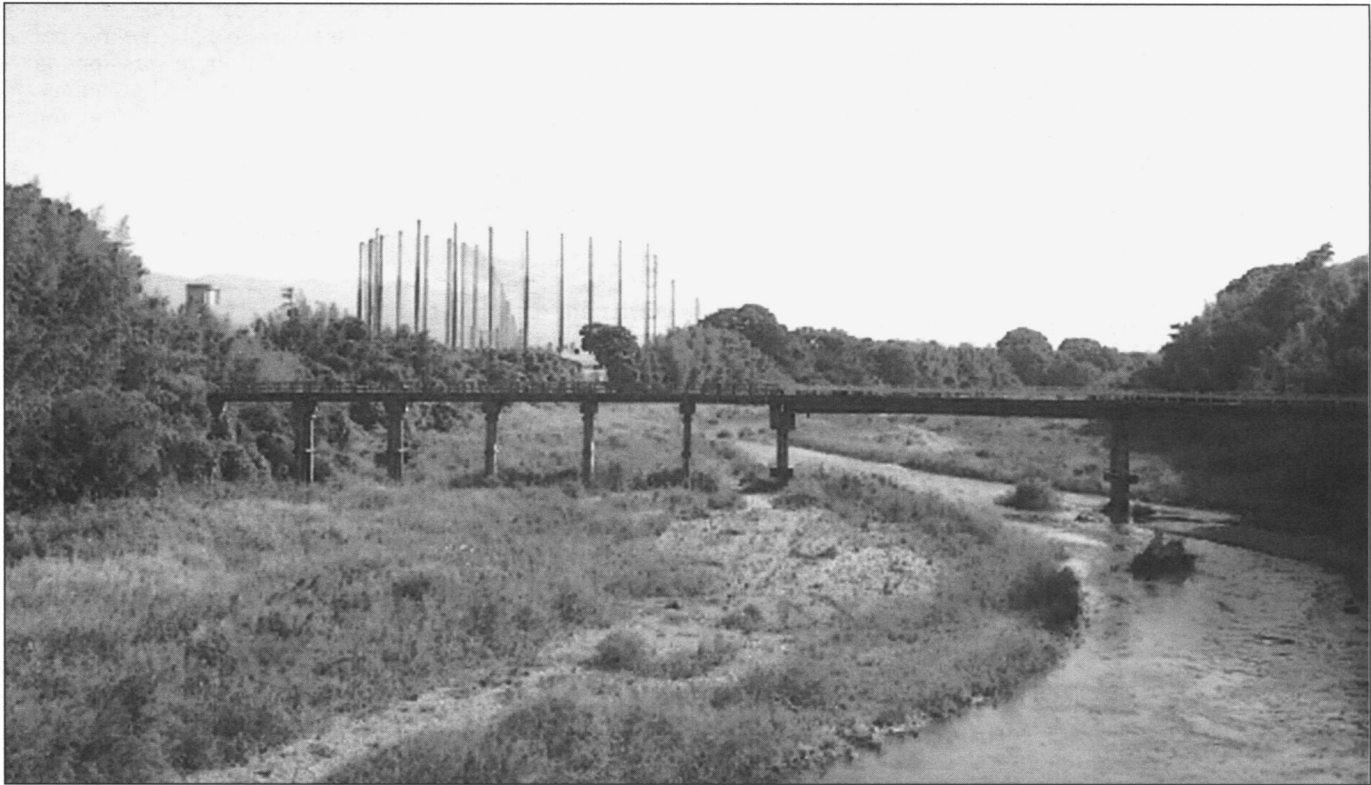
Fig. 1: The lower reaches of the Inukami river (Ima-bashi) – the right half fell, and was reconstructed.
