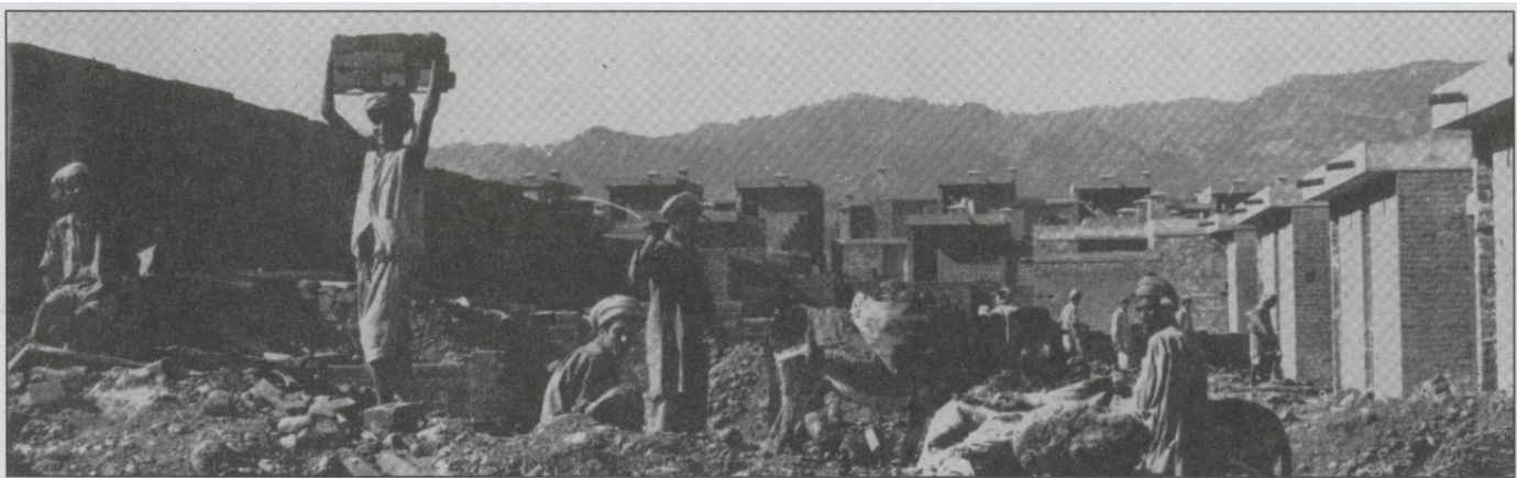
Fig. 35: First community of lower income housing under construction.
