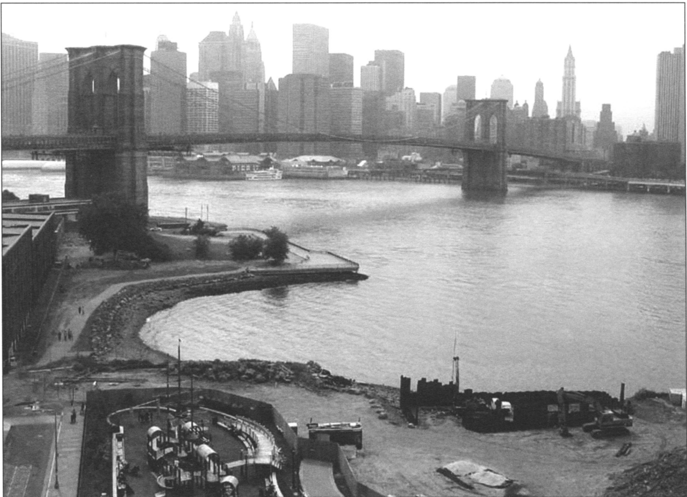
Fig. 2: The Brooklyn Bridge and port lands.
