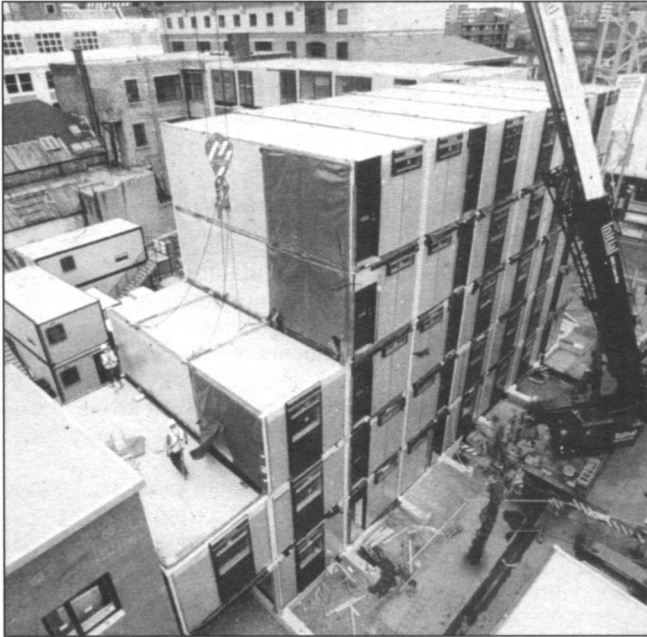
Fig. 1: A volumetric housing scheme under construction in London.
