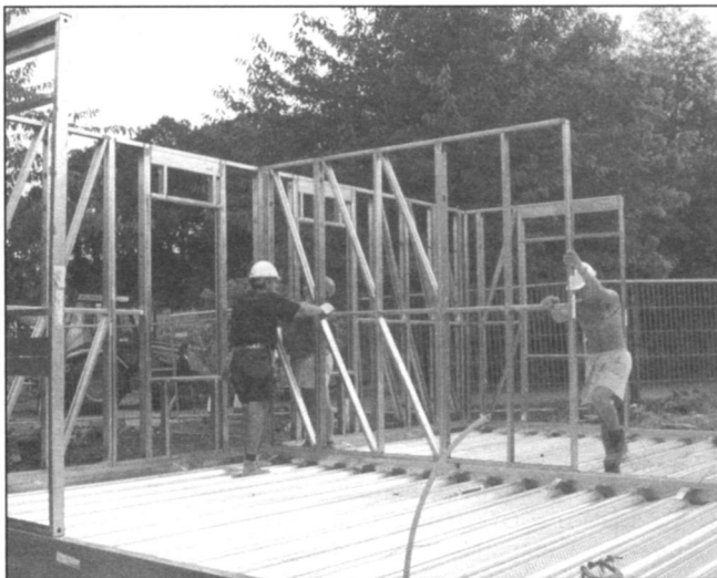
Fig. 2: Light steel frame panellized construction.
