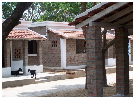
Fig. 1: Self-build dwellings, Artes-ISED-ADER-ISCOS project, Sirkazhi Taluk. Source: Balsavar
