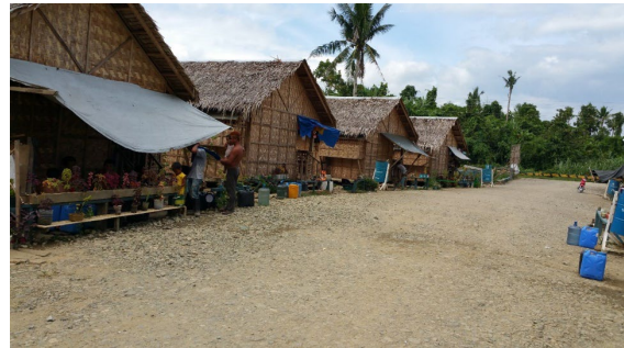
Fig.1: Temporary resettlement housing units Photo credit: Glenda Tibe Bonifacio, Tacloban City,
