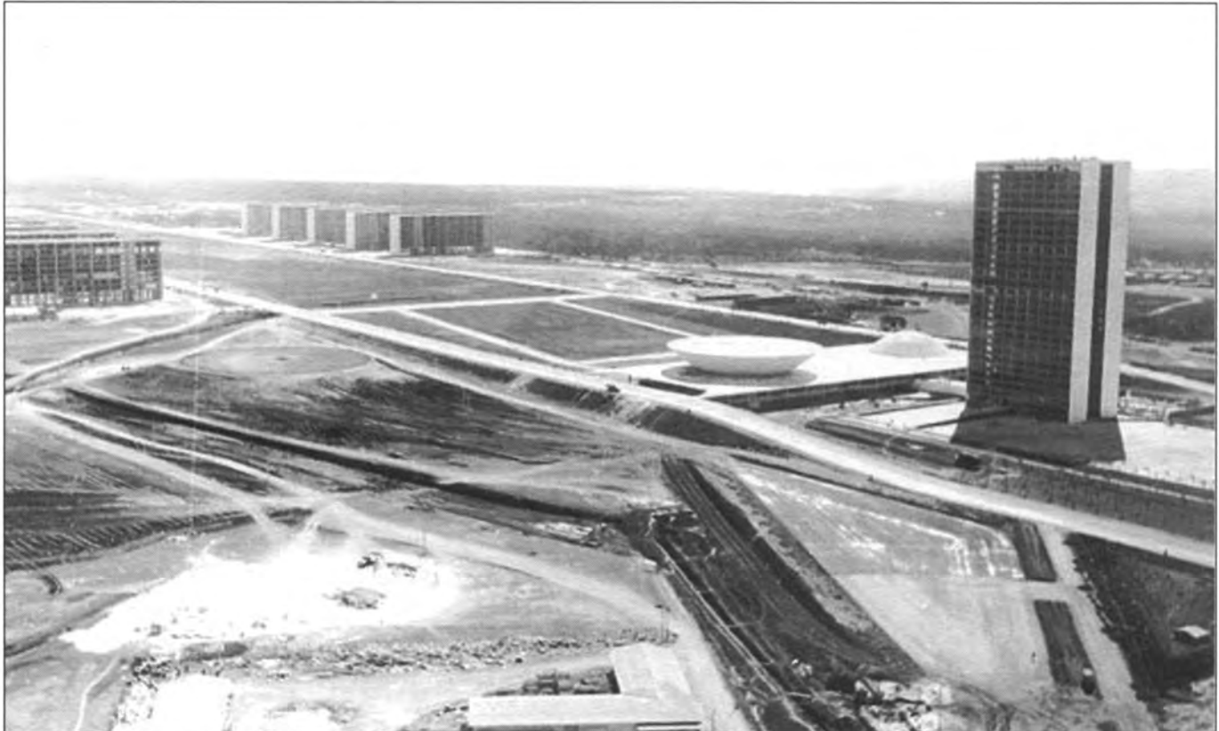
Fig. 3: Brasília – General view of Oscar Niemeyer's architectural synthesis: buildings of Brazilian Congress and Esplanade of the ministries during construction, circa 1960. (Source: © Arquivo Público do Distrito Federal, digitized by August Real).
