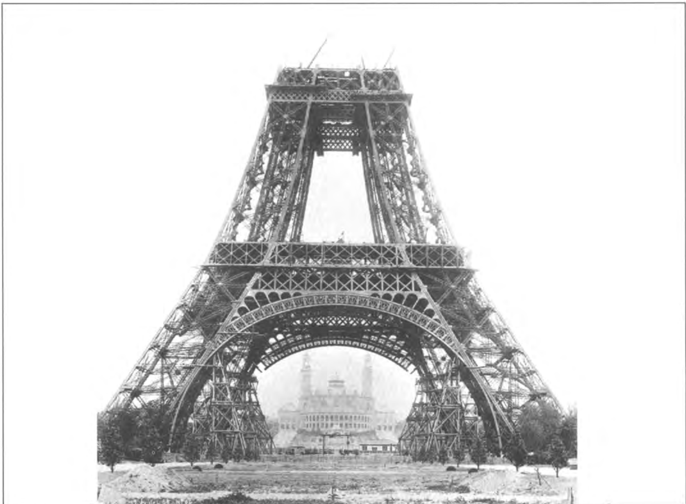
Fig. 7: Paris – The Trocadero Palace and the construction of the Eiffel Tower for the exhibition of 1889. (Source: Durandelle, Travaux de construction de la Tour Eiffel, 1888 . Paris, Editions Hazan, 1989).
