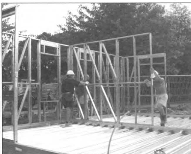
Fig. 2: Light steel frame panellized construction.
