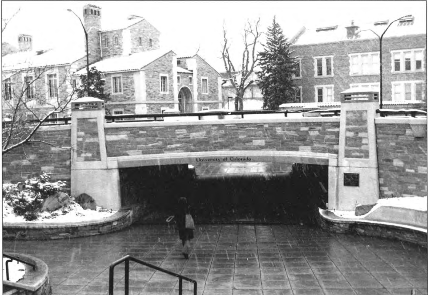
Fig. 3: Successful new towns and cities of the future will separate vehicular traffic from cyclists and pedestrians. This underpass improves mobility and safety, especially in wintry conditions. (Source: The author).
